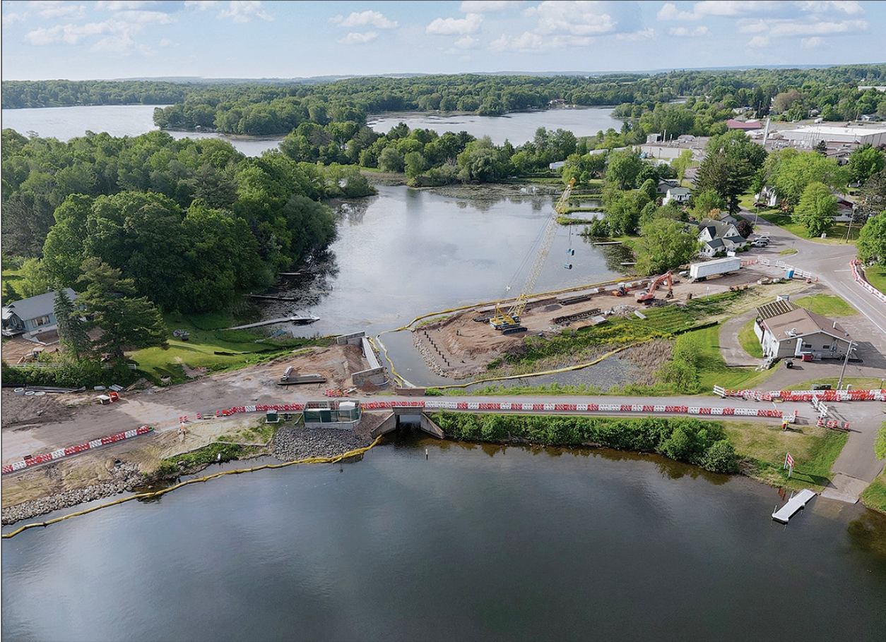
MARTY PETERS USED A DRONE TO SHOW THE HWY 63 BRIDGE PROJECT FROM ABOVE. WORK WILL CONTINUE THROUGHOUT THE SUMMER.
